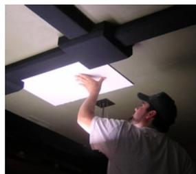
same three templates are used throughout to maintain uniform spacing. For flat ceilings, acoustic ceiling adhesive is used. Sloped ceilings will require additional screws or nails to prevent drift.
